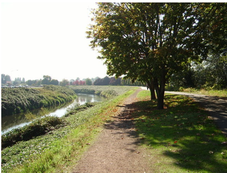
Photo 4-4. Green River Levee near Costco north of S. 180 th St.
