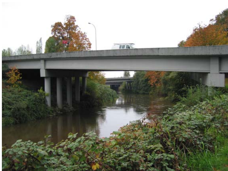
Photo 4-5. Bridges across Green River in Tukwila.
