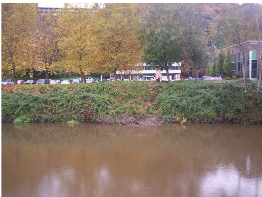
Photo 4-2. View of the left (west) bank of the Green/Duwamish River near RM 11.7 taken from the Green River trail on November 2, 2006.
