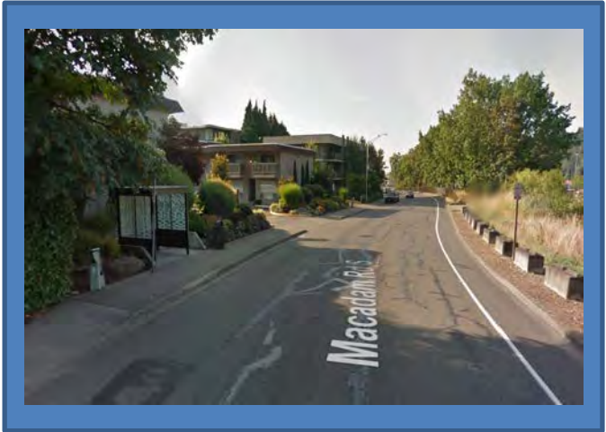
Macadam Rd S, showing existing sidewalk, bike lanes, curb, and concrete blocks; looking south
