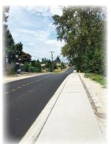
The project included upsizing and looping the undersized and dead-end water main along Macadam Road to improve capacity, fire flow, and redundancy. The project also added 1,200 feet of sidewalk on the east side, bridging the existing gap, and a full-width overlay (complete paving and striping of all lanes).
