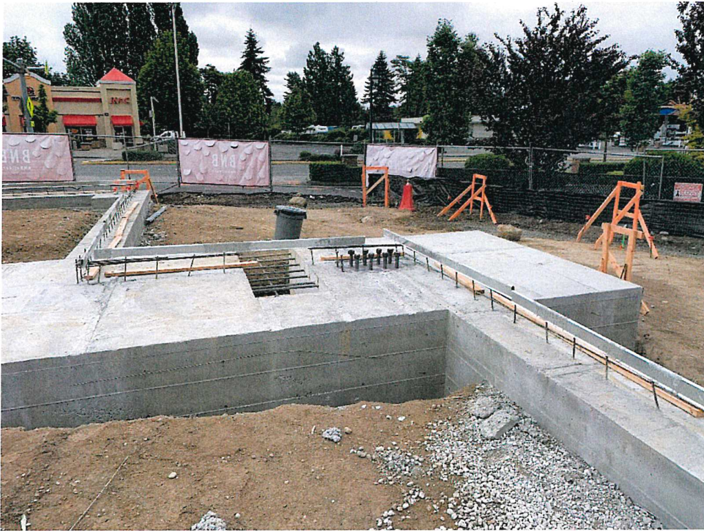
Concrete Footings Poured at South Lot
