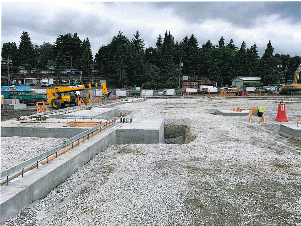
Concrete Footings Poured at South Lot
