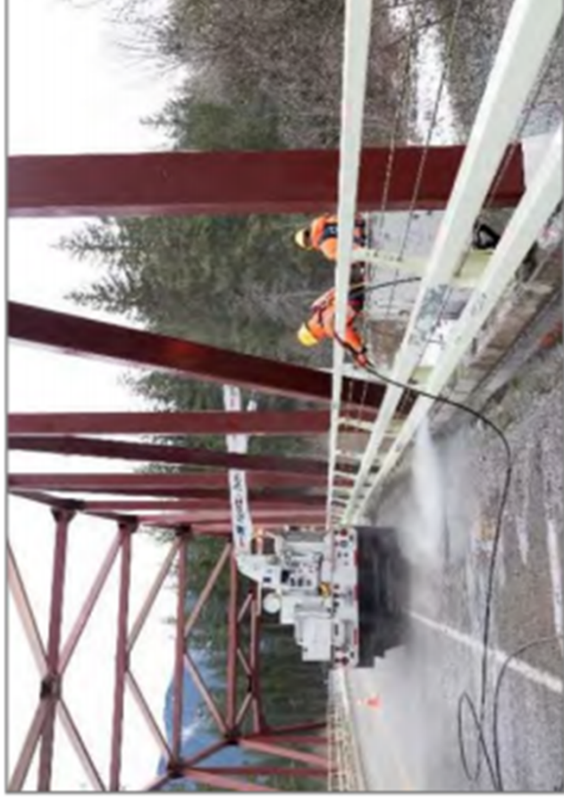
Mt. Si Bridge No. 2550A during bridge washing process.
