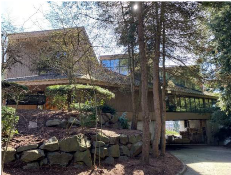
Figure 3.1-2. City Hall, West End (looking south).
