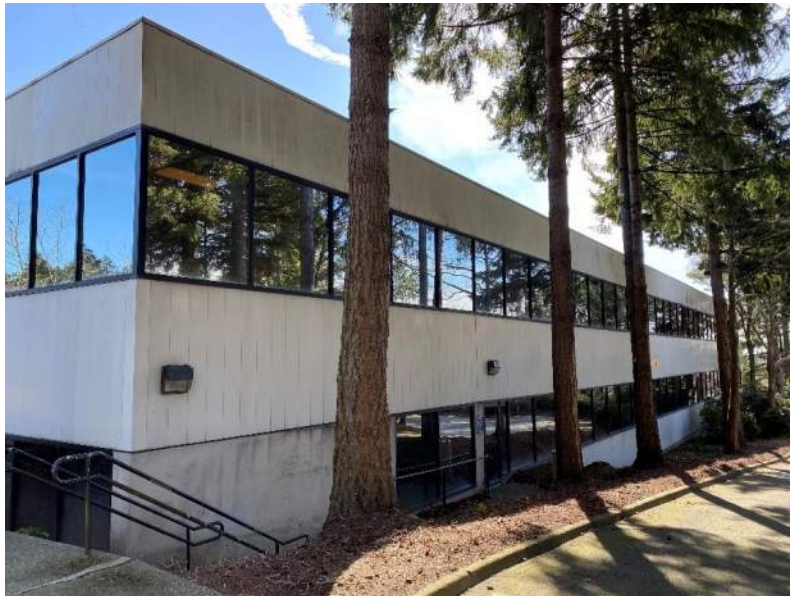
Figure 3.2-1. 6300 Building, West Exterior.
